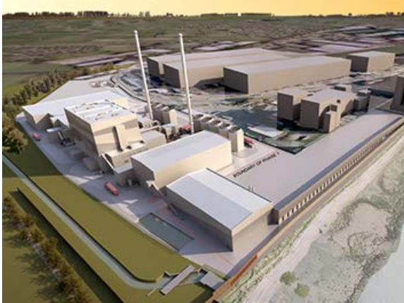
Tilbury Green Power, London, UK
